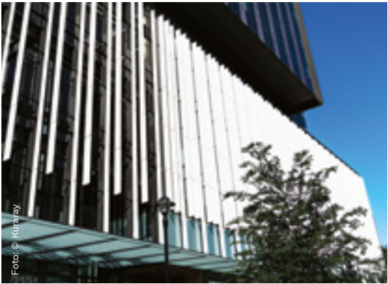
New Headquarters Building, Seattle, USA
