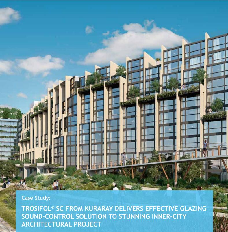
TROSIFOL® Sound Control (SC), a sound-attenuating PVB acoustic film from Kuraray, has given Marvel Architects the ability to incorporate a substantial glazed façade on a residential development, which would otherwise may not have been feasible due to localised noise levels from the surrounding locale.
