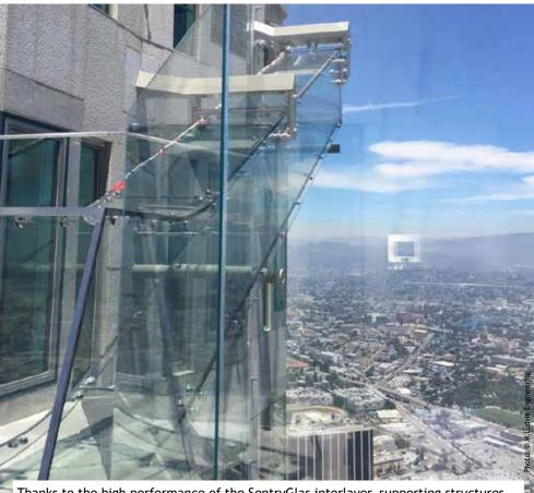
Thanks to the high performance of the SentryGlas interlayer, supporting structures are kept to a minimum leaving virtually unobstructed views of the LA skyline
