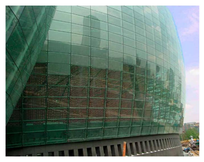
Andreu wanted a shimmering, glass-metal effect, which glowed beautifully at night. Laminated safety glass was a must for such a façade. However, PVB, the traditional bonding ingredient of laminated glass, does not adhere well to metal. The solution: SentryGlas® interlayer, which not only adheres to glass but creates an incredibly strong bond to metal as well.
