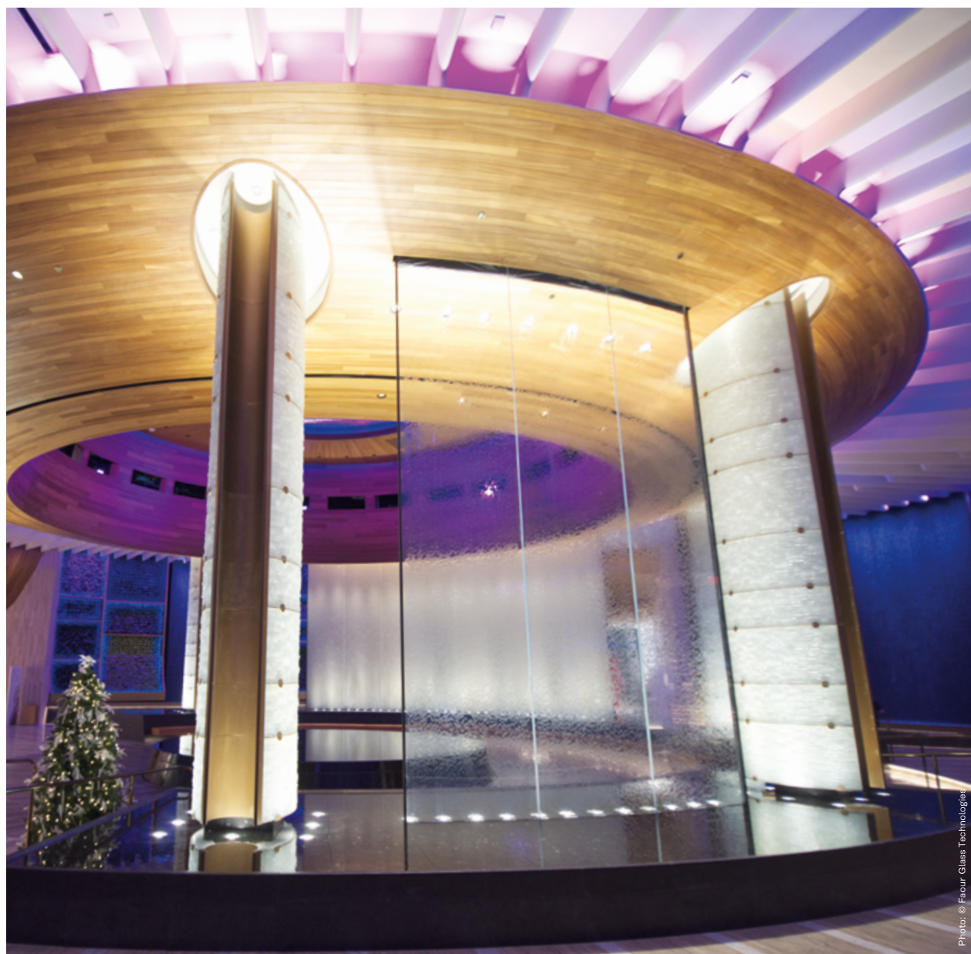
Based around a 12.2 m (40 ft) diameter glass cylinder, the Oculus comprises fourteen panels of custom-laminated glass, some with a projection film applied.
