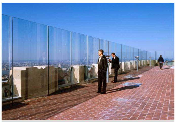
To meet wind loads and weathering requirements, the glass construction consists of two layers of 15 mm ( $^{19}/_{32}$  in.) lowiron laminated tempered glass with a 2.28 mm ( $^{90}$  mil) SentryGlas® interlayer.
