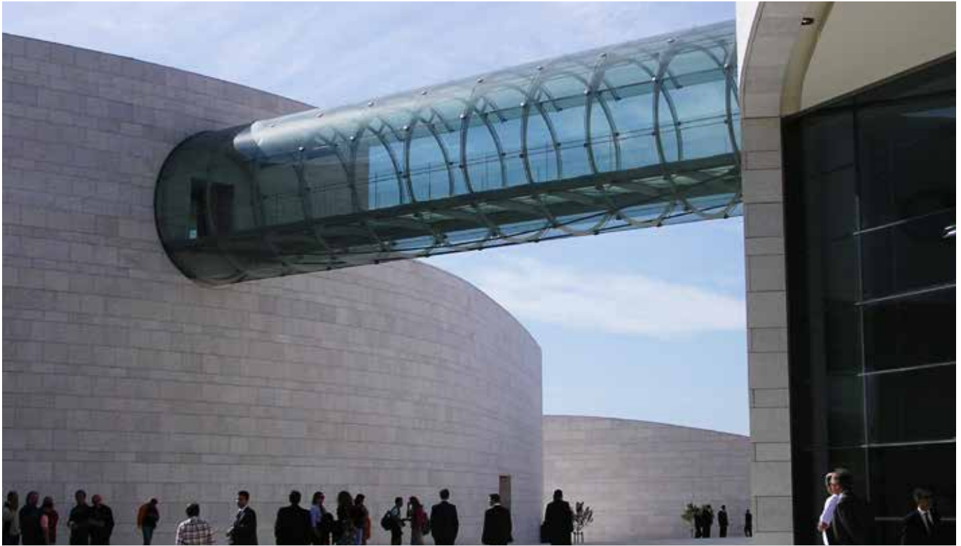
The two buildings at the ‘Champalimaud Centre for the Unknown’ are connected by a lightweight steel and glass bridge encased by curved panels of laminated glass made with SentryGlas® ionoplast interlayer. The stiff and strong high-performance interlayer from DuPont was specified for the installation on the basis of its decreased deflection and superior post breakage behaviour as compared to laminates made with PVB. Photo: Bellpart
