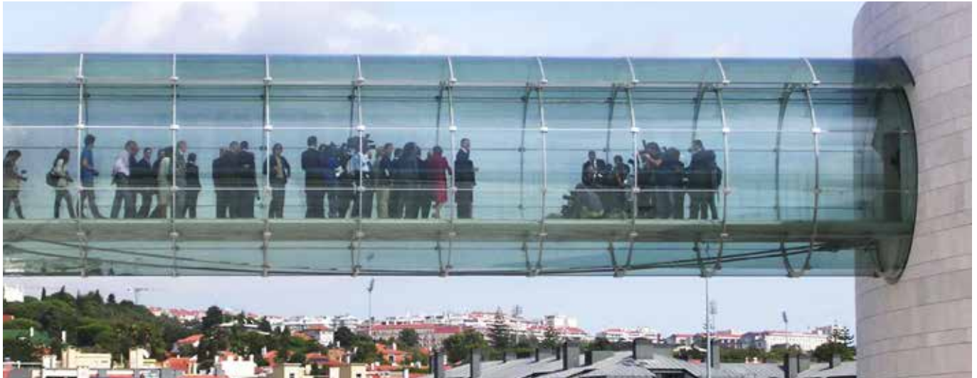
The curved glass envelope for the bridge consists of several laminated glass panels, each typically measuring 1950 x 1320 mm (78 x 52"), which are held in place by four custom-designed clamp plates located at the glass vertices. Vertical steel rings positioned at every two meters along the envelope are used for its support. Photo: Bellapart
