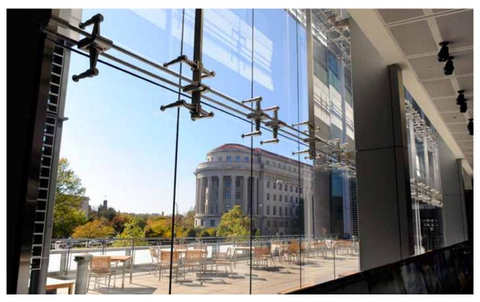
Moreover, SentryGlas® interlayer enhances the safety and strength of the entire assembly. Its post-break strength is higher than that of PVB, and it keeps glass in place even when shattered. The use of two layers of 10 mm (3/8 in.) low-iron tempered glass laminated with 1.52 mm (60 mil) SentryGlas® allowed Polshek partnership to achieve its transparent "window on the world."
