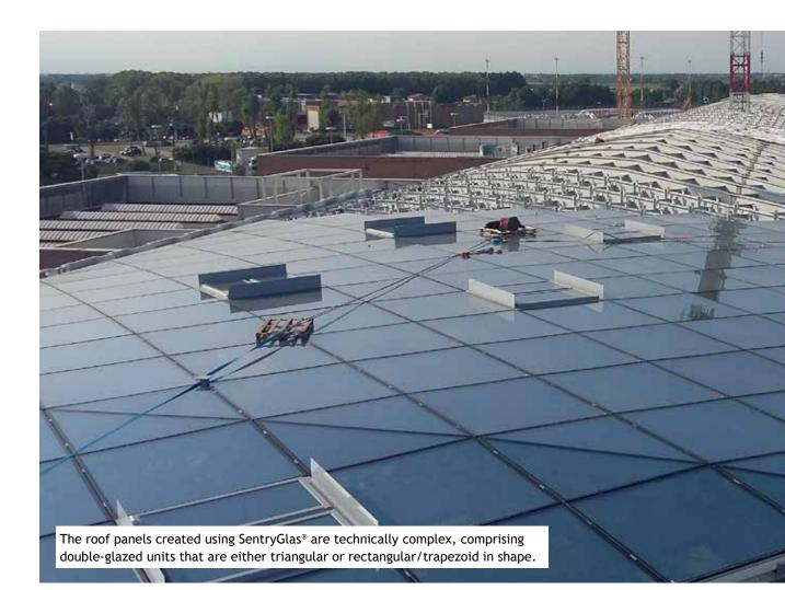
According to Roberto Arias, marketing manager at Tvitec, the glass fabricator: "The roof panels created using SentryGlas<sup>®</sup> ionoplast interlayers from Trosifol are really technically complex. They comprise doubleglazed units that are either triangular or rectangular/ trapezoid in shape, most of which are over 2 m (6 ft) in size."
