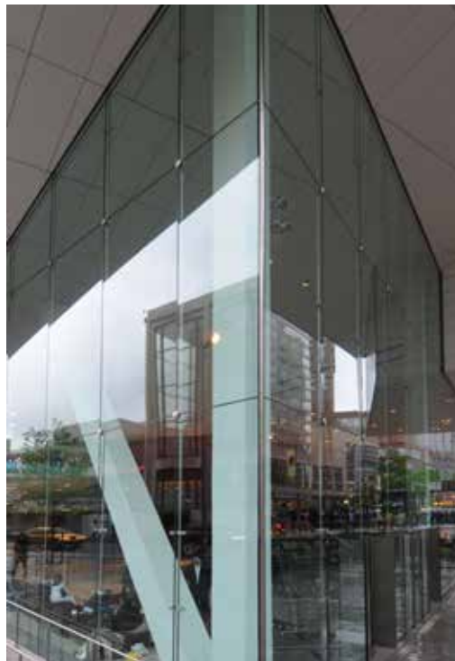
SentryGlas® helped W&W Glass engineer a frameless leading edge for the Alice Tully Hall renovation, adding to its feeling of openness.
