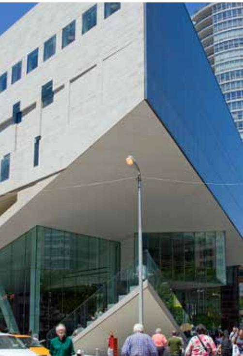
SentryGlas® helped W&W Glass engineer a frameless leading edge for the Alice Tully Hall renovation, adding to its feeling of openness.
