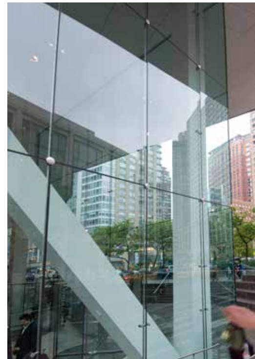
SentryGlas® helped W&W Glass engineer a frameless leading edge for the Alice Tully Hall renovation, adding to its feeling of openness.
