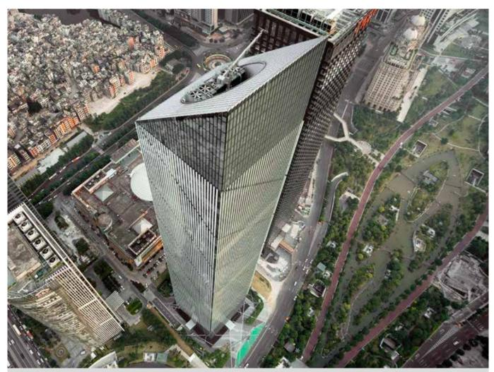
At 303 m (994 ft), the Leatop Plaza is Guangzhou's fifth tallest building. Of the total façade area of 159,500 m<sup>2</sup> (1.700.00 sq ft), SentryGlas® was used over 63,000 m<sup>2</sup> (678.000 sq ft), for its strength and energy-saving capabilities.
