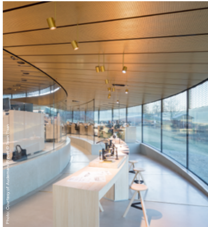
• The load-bearing curved glass panels are triple glazed and are affixed using structural silicone to geometrically bed them into steel shoes.
