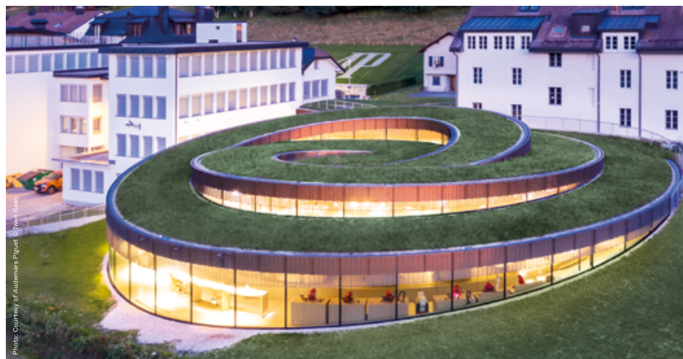
• When viewed from above, the structure – the first of its kind to be built at such altitude – resembles a watch spring and comprises two interlocking spirals, separated by glazed panels, looping around a common centre.
