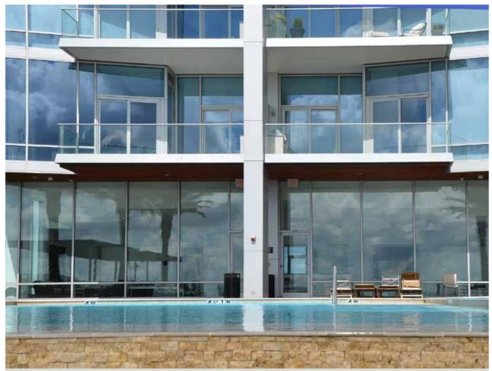
The frameless glass railing system installed at 2727 Kirby Drive, a 30-storey luxury condominium tower block in Houston, Texas. 143 balconies were retrofitted with C.R. Laurence's patented CRL L56S Series TAPER-LOC® Glass Railing System and SentryGlas® ionoplast interlayers.
