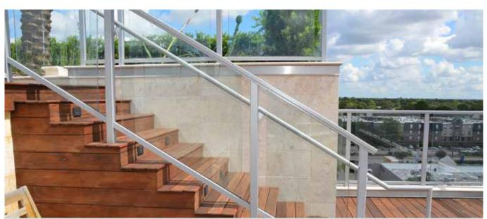
CRL's 200 Series ARS Aluminum Railing System was retrofitted to the pool deck areas at Kirby Drive. SentryGlas® was chosen because it is safer and stronger than alternative laminates and is extremely clear, giving residents virtually crystal clear, unobstructed views from their balconies. SentryGlas® also offers excellent weathering durability with no discolouration, creep or delamination issues.
