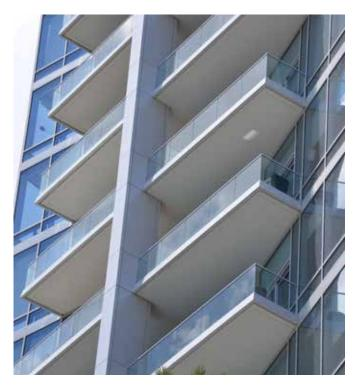
SentryGlas® is more than 100 times stiffer and 50 percent stronger than PVB alternatives. Due to the strength of the interlayer, SentryGlas® demonstrate excellent postglass-breakage performance. Upon impact, the glass may break, but dangerous fragments will adhere to the SentryGlas® interlayer, reducing the risk of injury to people in the vicinity.
