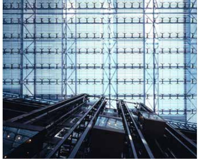
The glass panels, which vary in shape and size all feature a three-layer construction comprising 8 mm (5/16 inch) heat-soaked fully-tempered SLS glass top and bottom plies, sandwiching a 2.28 mm (90 mil) SentryGlas® interlayer.
