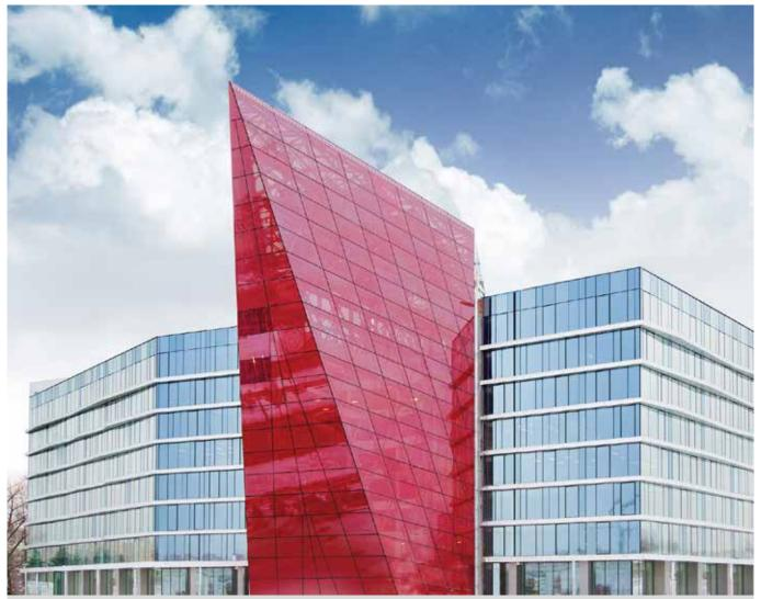
The red crystal structure at the centre deploys SEFAR® Architecture VISION fabric AL 260/55 printed, which gives glass a textile-like structural quality.
