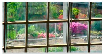
Double-glazed, insulated glass panels address safety requirements and plant health needs.
