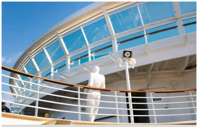
To meet wind loads and weathering requirements, the glass construction consists of two layers of 15 mm (19/32 in.) low-iron laminated tempered glass with a 2.28 mm (90 mil) SentryGlas® interlayer.
