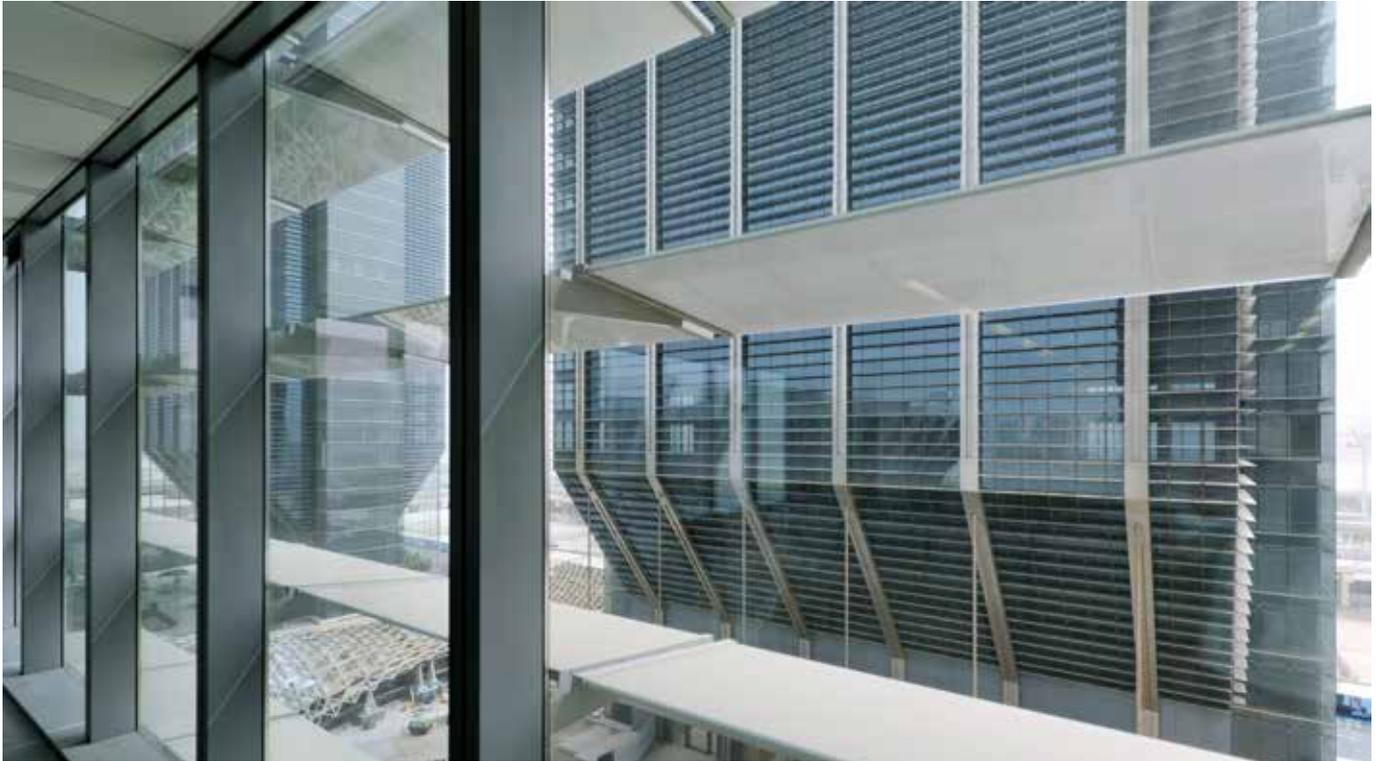
*Constructed by German laminator BGT, the laminate glass panels used for the louvers were decorated with a special silk screen printed, two-colour congruent pattern in order to minimise the G-value. SentryGlas® was selected for its resistance to humidity and high temperatures, as well as its post-breakage behaviour and open edge performance.*
