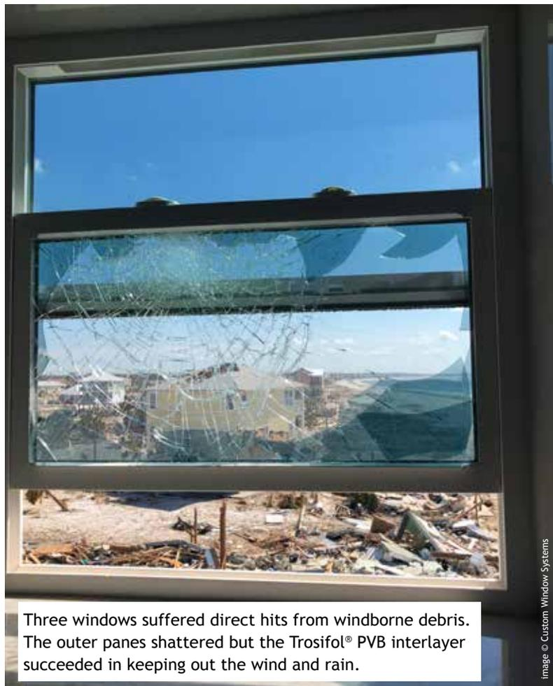
Three windows suffered direct hits from windborne debris. The outer panes shattered but the Trosifol® PVB interlayer succeeded in keeping out the wind and rain.
