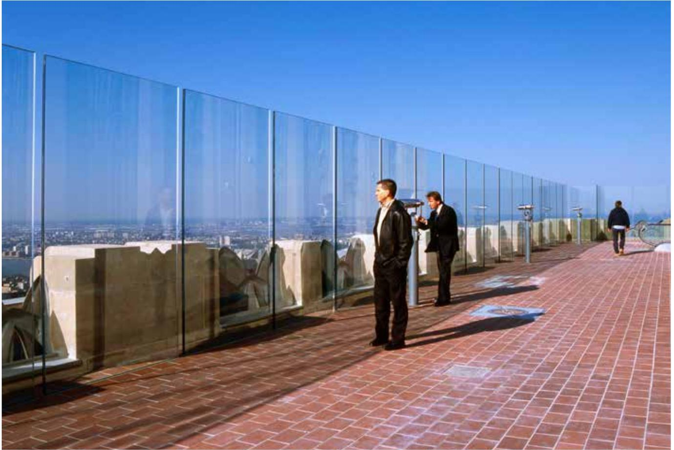
*To meet wind loads and weathering requirements, the glass construction consists of two layers of 15 mm (19/32 in.) low-iron laminated tempered glass with a 2.28 mm (90 mil) SentryGlas® interlayer.*
