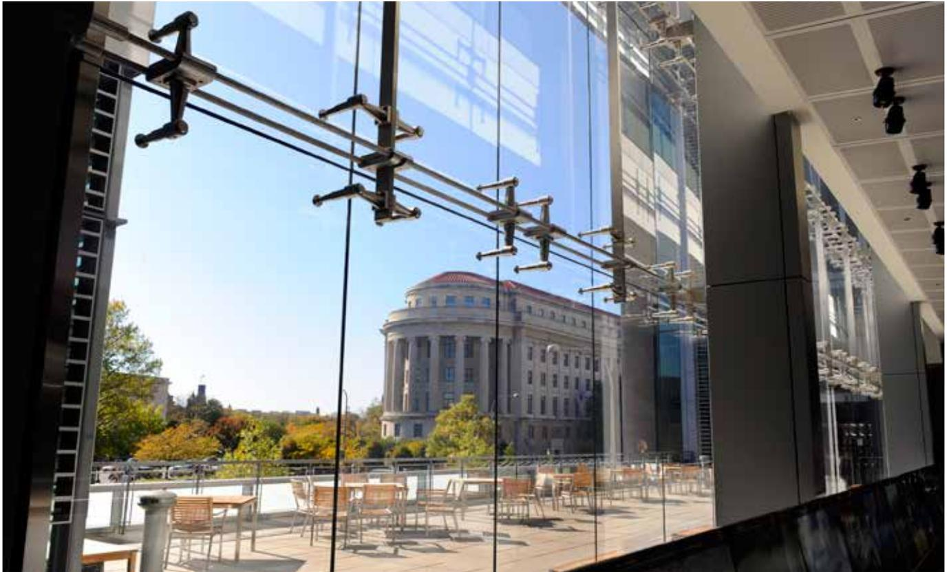
Moreover, SentryGlas® interlayer enhances the safety and strength of the entire assembly. Its post-break strength is higher than that of PVB, and it keeps glass in place even when shattered. The use of two layers of 10 mm (3/8 in.) low-iron tempered glass laminated with 1.52 mm (60 mil) SentryGlas® allowed Polshek partnership to achieve its transparent "window on the world."
