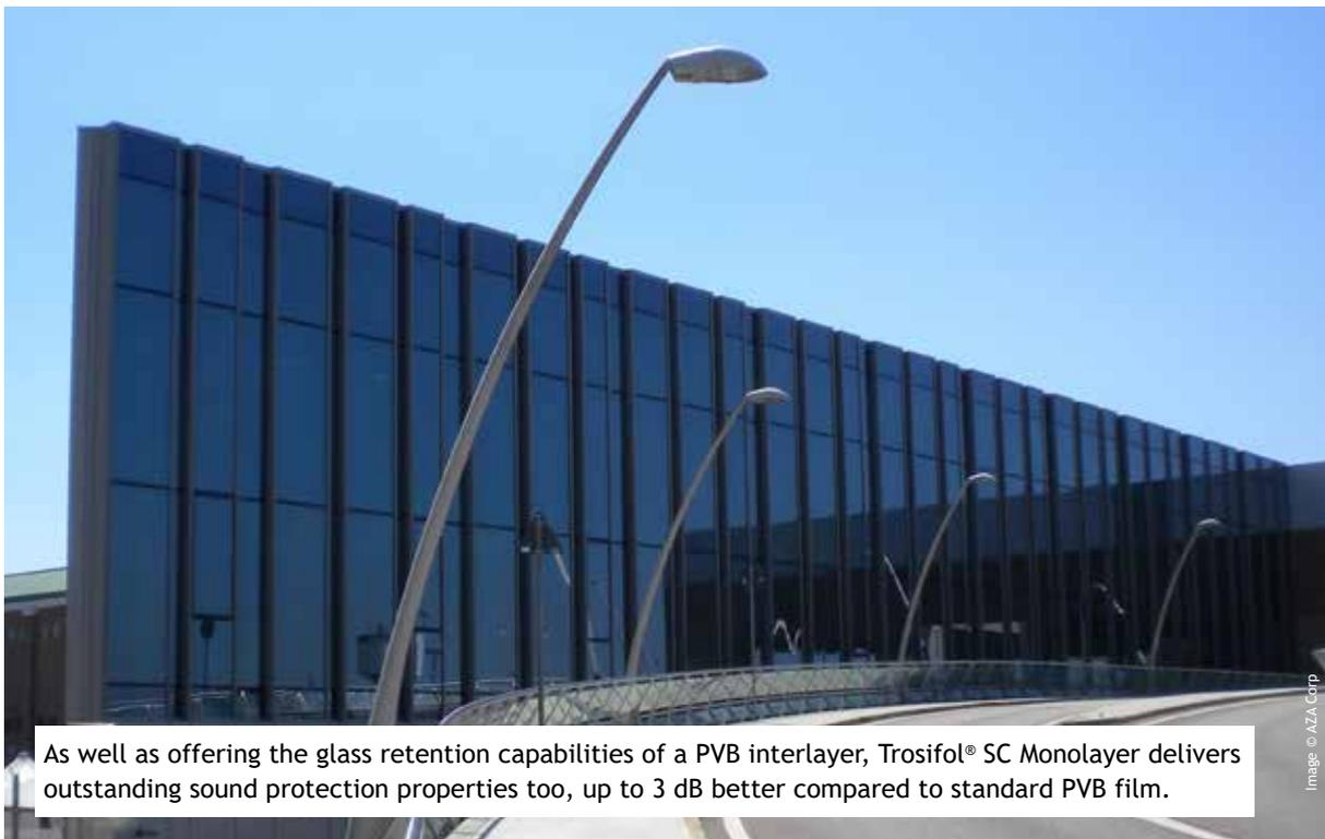
As well as offering the glass retention capabilities of a PVB interlayer, Trosifol® SC Monolayer delivers outstanding sound protection properties too, up to 3 dB better compared to standard PVB film.
