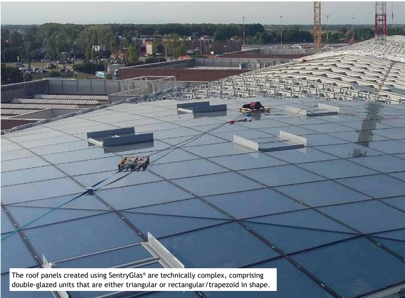
The roof panels created using SentryGlas® are technically complex, comprising double-glazed units that are either triangular or rectangular/trapezoid in shape.
