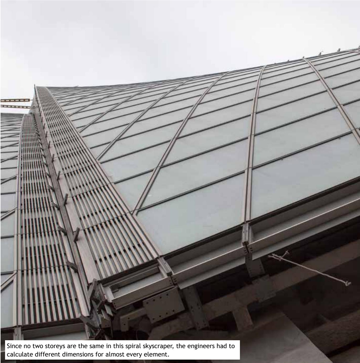
Since no two storeys are the same in this spiral skyscraper, the engineers had to calculate different dimensions for almost every element.
