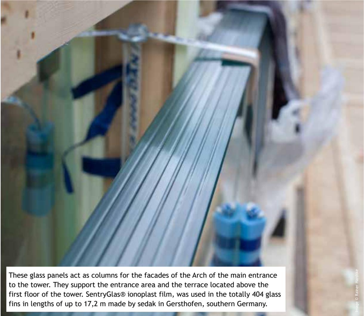
These glass panels act as columns for the facades of the Arch of the main entrance to the tower. They support the entrance area and the terrace located above the first floor of the tower. SentryGlas® ionoplast film, was used in the totally 404 glass fins in lengths of up to 17,2 m made by sedak in Gersthofen, southern Germany.
