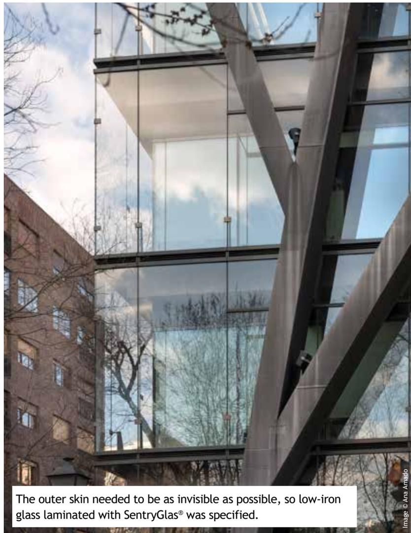
The outer skin needed to be as invisible as possible, so low-iron glass laminated with SentryGlas® was specified.
