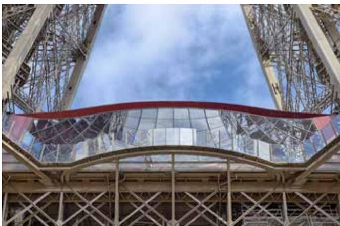
“Weight of the glass was also limited by the structure itself. PVB interlayers were considered, but these could not give us the weight [glass thickness] reduction that we required for the first floor project. We also needed to preserve the transparency of the glass floor and balustrades, which again pointed to the use of SentryGlas® interlayer,” continued Guitart.
