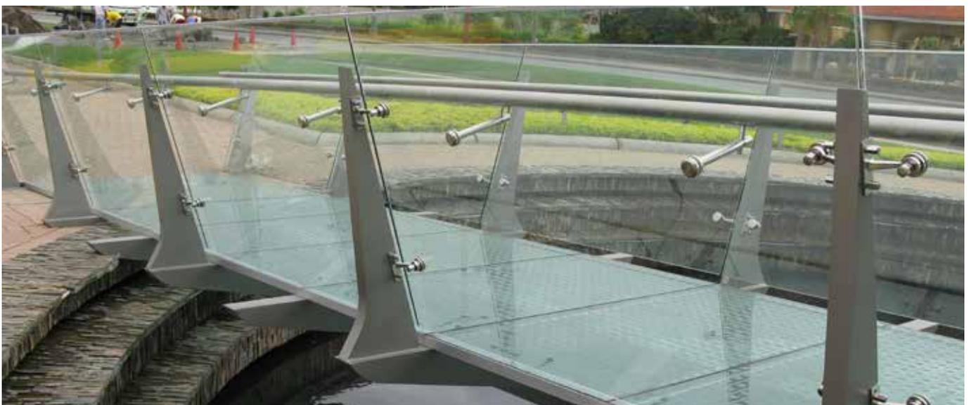
*SentryGlas® was also used on a 14m (approx. 46 ft) walkway that forms the entrance to the building. The walkway comprises three tempered glass panels with 1.52 mm (60 mil) SentryGlas® interlayers.*
