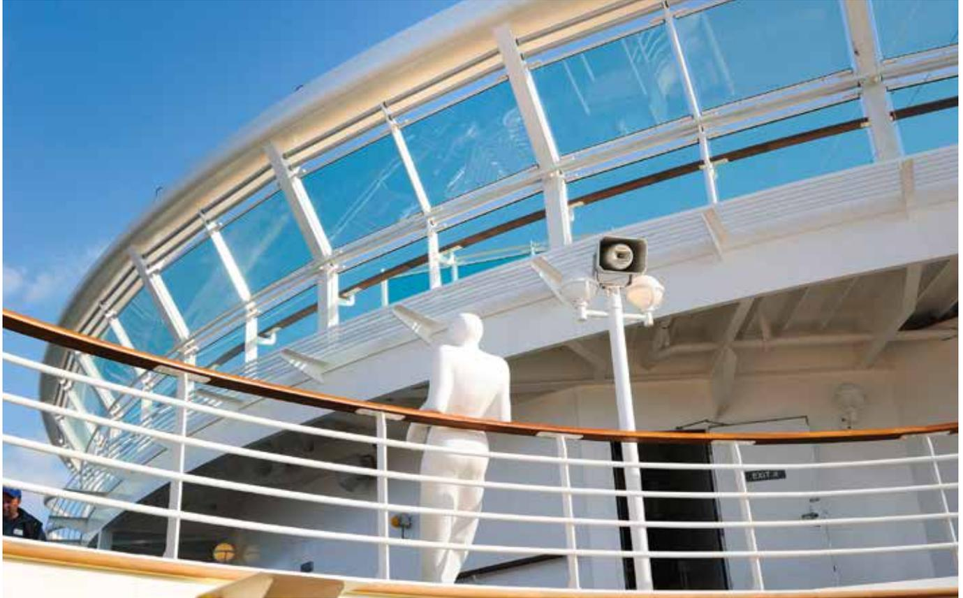
*To meet wind loads and weathering requirements, the glass construction consists of two layers of 15 mm (19/32 in.) low-iron laminated tempered glass with a 2.28 mm (90 mil) SentryGlas® interlayer.*
