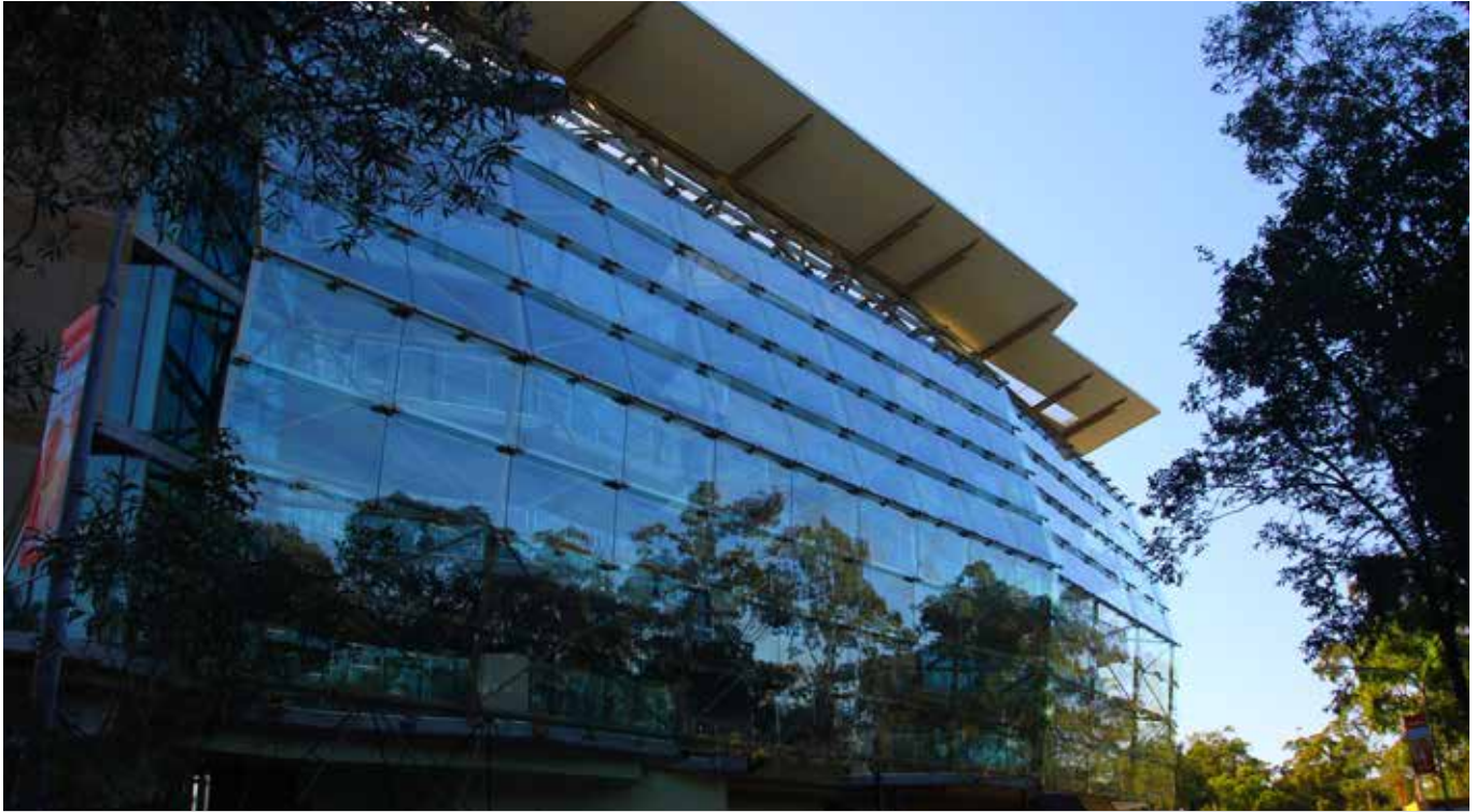
The building's south-facing side features a bowed glass façade set out from the building as a 'rain-shield' that allows circulation edges to be naturally ventilated.
