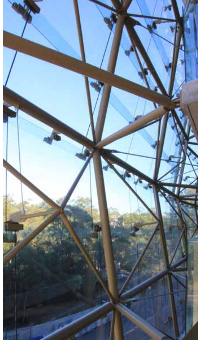
The use of a SentryGlas® ionoplast interlayer offered the thinnest and subsequently the lightest design for this feature screen using heat strengthened laminated glass.
