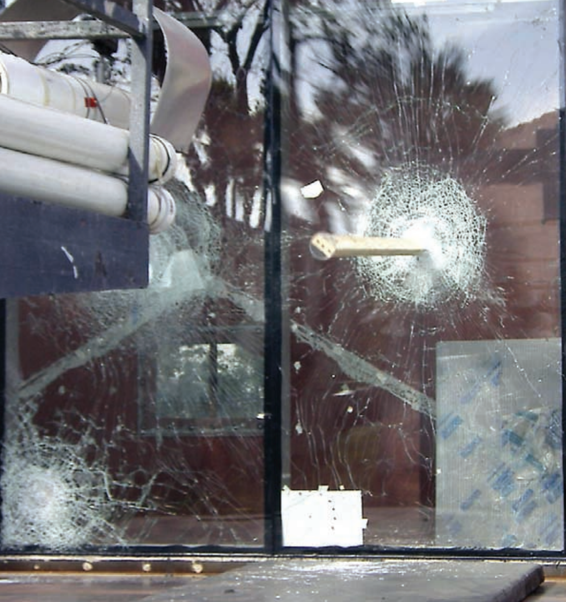
Typical impact test of a four-sided structural glazed unit.
